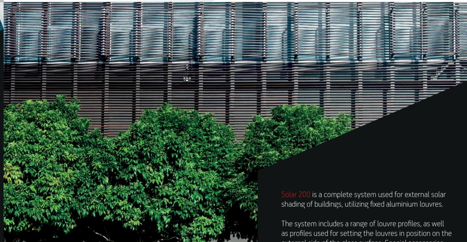
**Solar 200** is a complete system used for external solar shading of buildings, utilizing fixed aluminium louvres.
